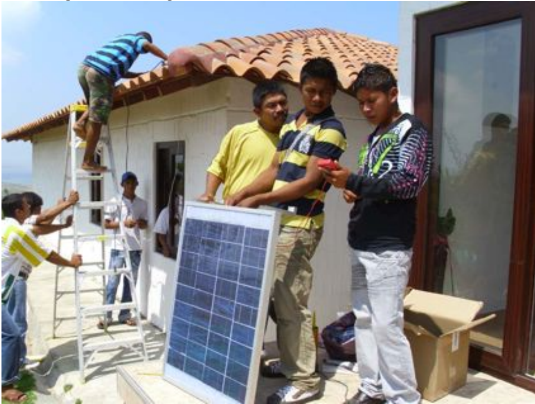
Checking the 65 watt PV module before installation on the roof
