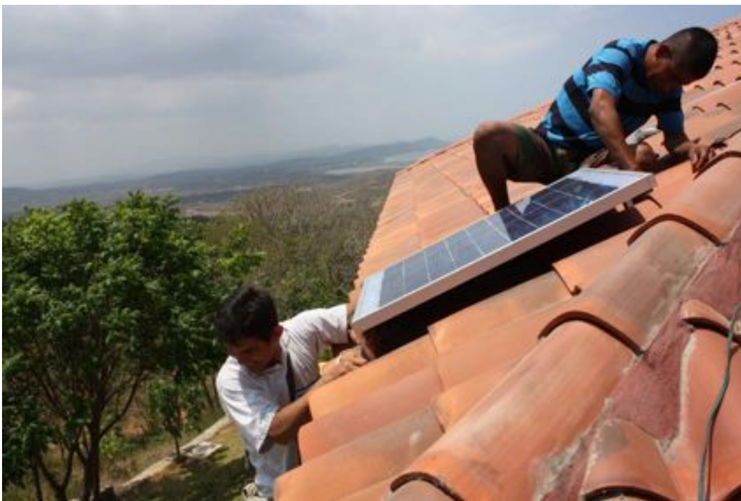
Finishing the installation
